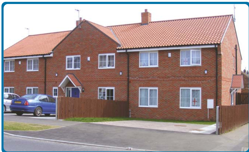
Homes at Eastfield in Scarborough
