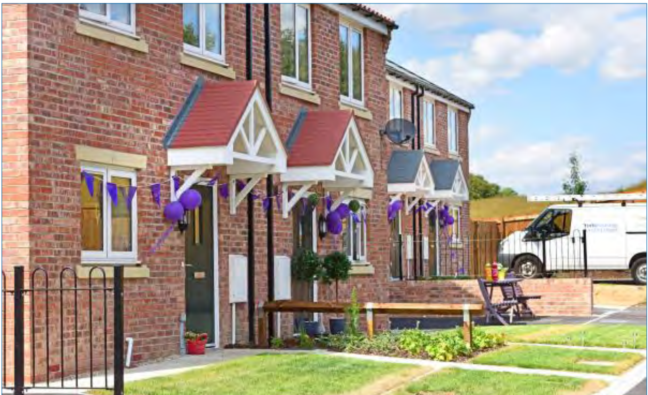
Rural Exception Site in Sheriff Hutton, Ryedale, completed by York Housing Association 2018
